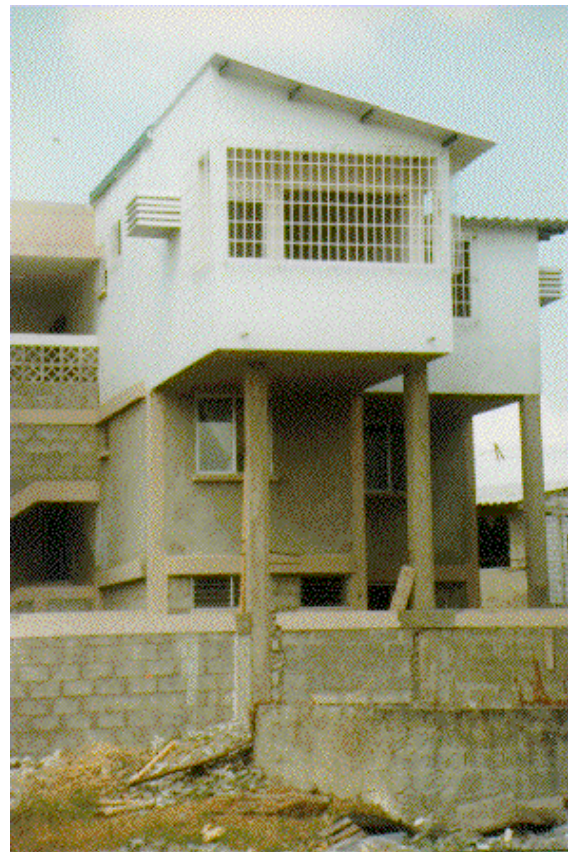
A type of structure with a high seismic risk are those condominiums built by BEV in Sauces IX, in which extensions have been built without any structural design and technical supervision. (Taken from the archives of IIFIUC - Universidad Católica, Project FUNDACYT-BID).
